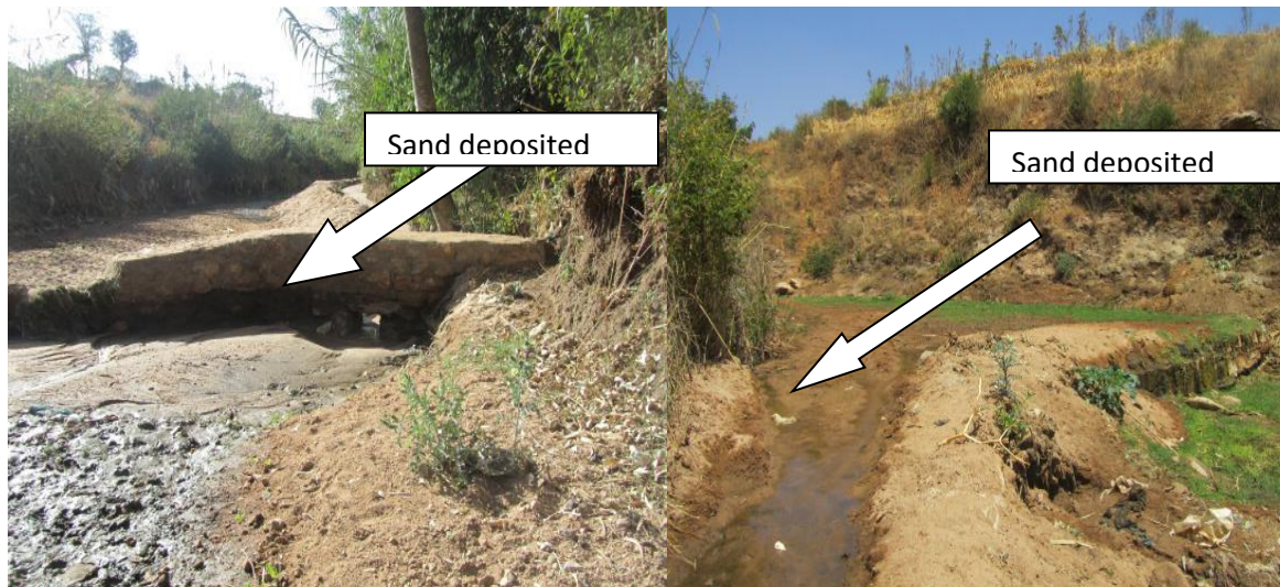
Figure 1: thick transported sand deposit at Mawir-I weir (left picture) and Mawir-II weir (right picture) sites
